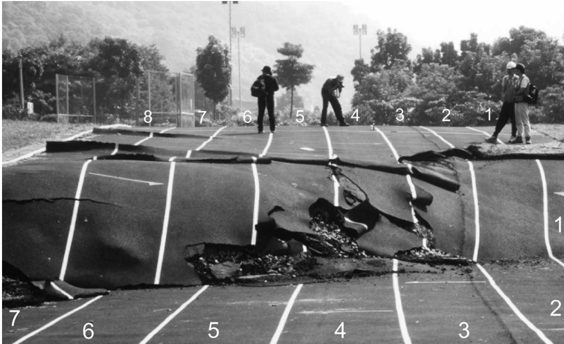
Fig. 7. Photograph of fault scarp of the September 21st earthquake, 1999, at sub-site B. Location in Fig. 4. View towards E, from footwall towards hanging wall. Stadium tracks numbered 1–8. Note the apparent right-lateral displacement of painted lines separating tracks, despite a left-lateral slip component (compare with map of sub-site B in Fig 4c; also see Fig. 9c). Same situation as in Fig. 6c, except for benchmark trend (E–W) and fault strike (NW–SE).
