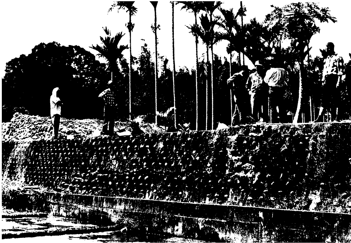
Fig. 13. The upper reverse fault in the Chinyuan channel, upstream subsite (site 5, northern Chinyuan village, location in Fig. 8b). Eastern side of the channel. SSE on right side. Wall built in 1984–1985, striking NNW–SSE and facing west, and 2–2.5 m high. Note that the reverse fault locally developed horizontally along a weak zone of aligned water drainage pipes in the wall. Note also that the fault ends to the left in a triangular zone, as discussed in text.
