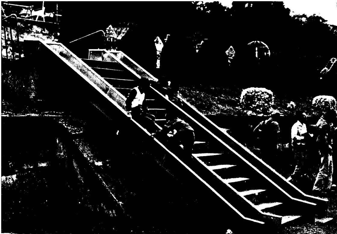
Fig. 9. The stairs of the Tapo school garden (site 2, location in Fig. 8b). View towards the SE. Note the uplift of the concrete block attached to the upper extremity of concrete stairs, as a response to shortening between Coastal Range (the garden, upstairs) and Longitudinal Valley (downstairs). Note also the concrete reinforcement added in the wall deformed by fault movement. Discussion of significance in text.
