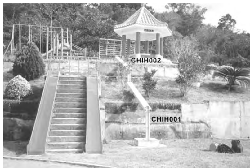
Figure 6. Photograph of the rod-type creep meter. The creep meters CHIH001 (the lower one) and CHIH002, with a common pier in the middle, cross the active fault zone and are aligned nearly perpendicular to the fault strike at the foot of rugged hills of the Coastal Range at the Tapo School.
